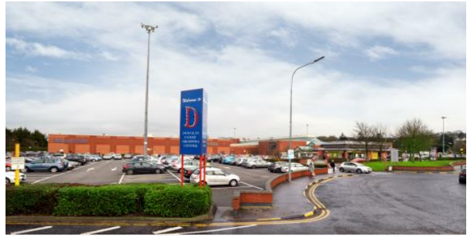
Douglas Court Shopping Centre, Douglas, Co. Cork
