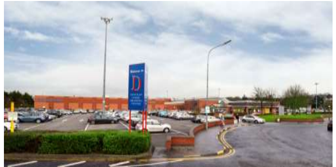
Douglas Court Shopping Centre, Douglas, Co. Cork
