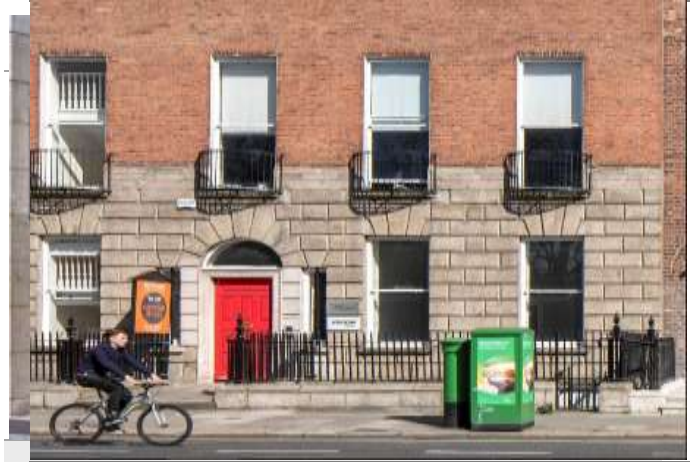
Second Floor, 28 Merrion Square, Dublin 2
