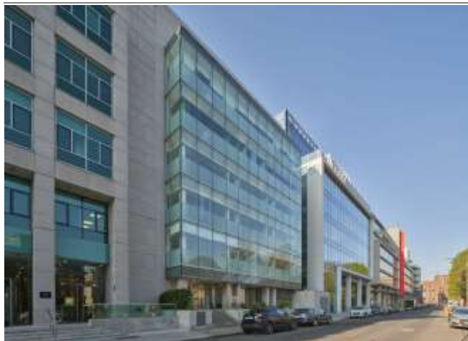
First Floor No.1 Hatch Street, Dublin 2
