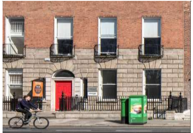
Second Floor, 28 Merrion Square, Dublin 2
