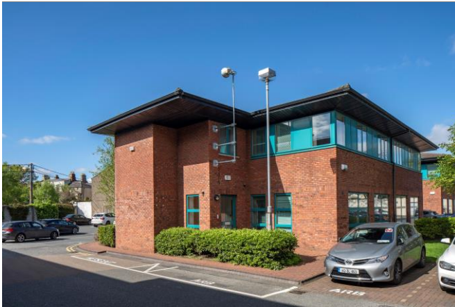
Block 9 Blackrock Business Park, Carysfort Avenue, Blackrock, Co. Dublin
