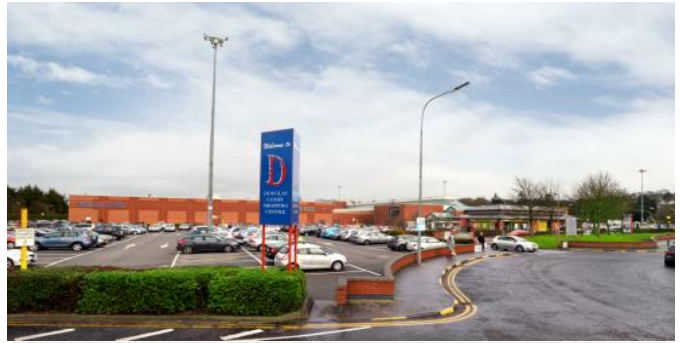
Douglas Court Shopping Centre, Douglas, Co. Cork
