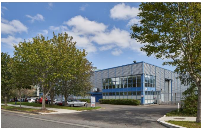
77 Furze Road, Sandyford, Dublin 18
