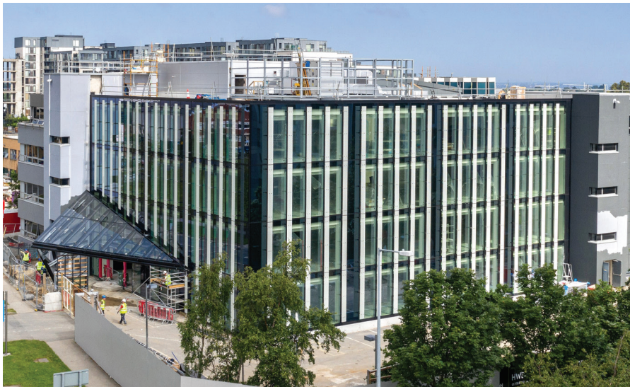
The HIVE Sandyford, Carmenhall Road, Sandyford, D18 New Grade A Offices 73,000 sq ft
