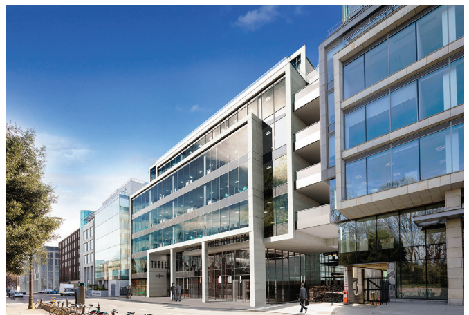
Three Park Place, Upper Hatch Street, Dublin 2. 30,000 sq ft acquired for Deloitte
