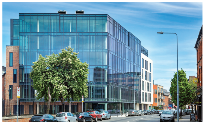
The Sharp Building, Hogan Place, Dublin 2. New Office HQ 45,000 sq ft let to Perrigo Pharma and sold to Credit Suisse
