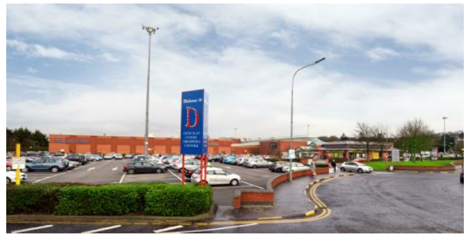
Douglas Court Shopping Centre, Douglas, Co. Cork
