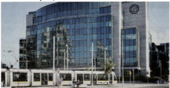
La Touche House, Dublin 1
