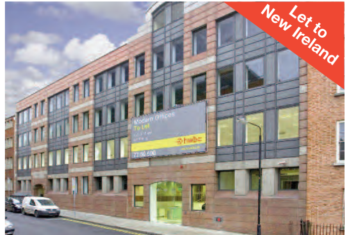
5/9 South Frederick Street, Dublin 2. Refurbished offices - 2,130 sq.m
