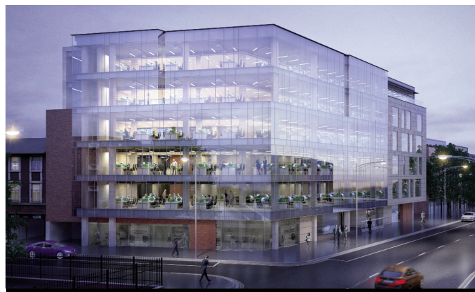
The Sharp Building, Hogan Place D2. New HQ under construction – 4,200 sq.m
