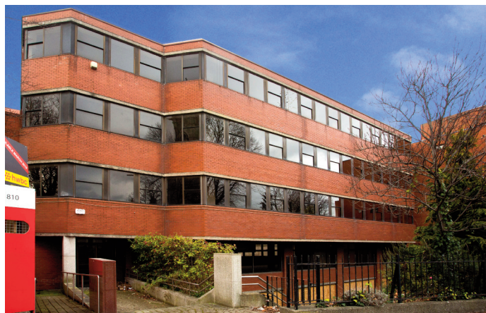
Haddington Court, Haddington Road, D4. High level refurb – 2,650 sq.m
